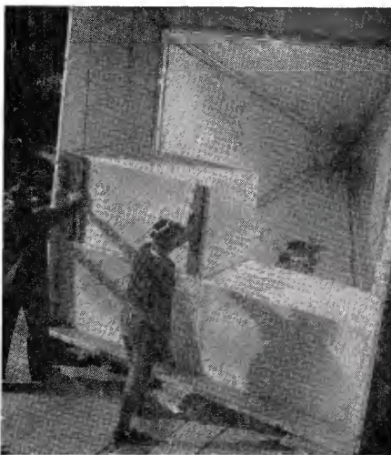
FIG. 8. ANTENNA IS ASSEMBLED AT TOWER SITE
