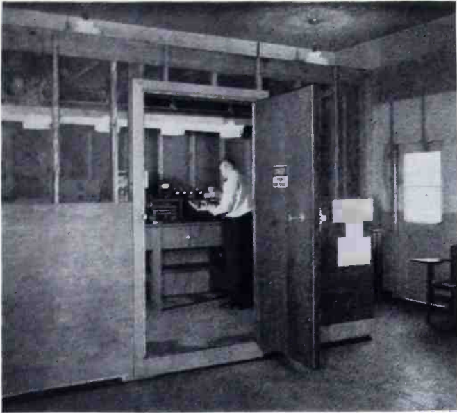
FIGS. 14 & 15. MAINTENANCE AND TEST ROOM AT LOS ANGELES HEADQUARTERS IS SURROUNDED COMPLETELY BY 2 INSULATED LAYERS OF SCREENING
