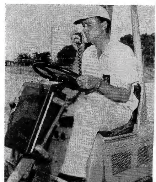
BELOW , Consolidated Vultee estimates that $30,000 a year will be saved by installing 2-way Motorola radio units on lift trucks and other vehicles at their Fort Worth plant, where B36D bombers are built.
