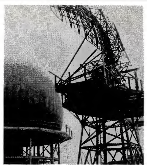
ABOVE , the balloon-like construction at the left is an Arctic Bubble, designed to protect a radar antenna of the type shown at the right from damage by the elements. The bubble, supported by internal air pressure, was photographed at the Bendix radar test site, near Baltimore, Md. This type of protection was developed particularly for service under sub-zero conditions where radar stations are operated by the U.S. Air Force and the Navy.
