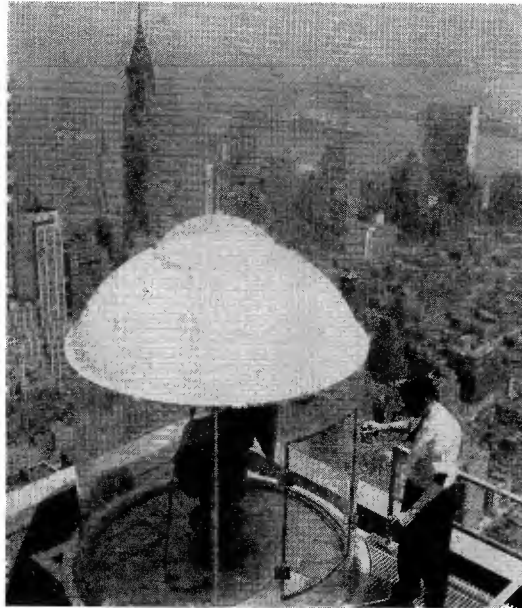
BELOW , an RCA microwave TV link mounted at the base of the new tower on the Empire State Building, facing northeast.
