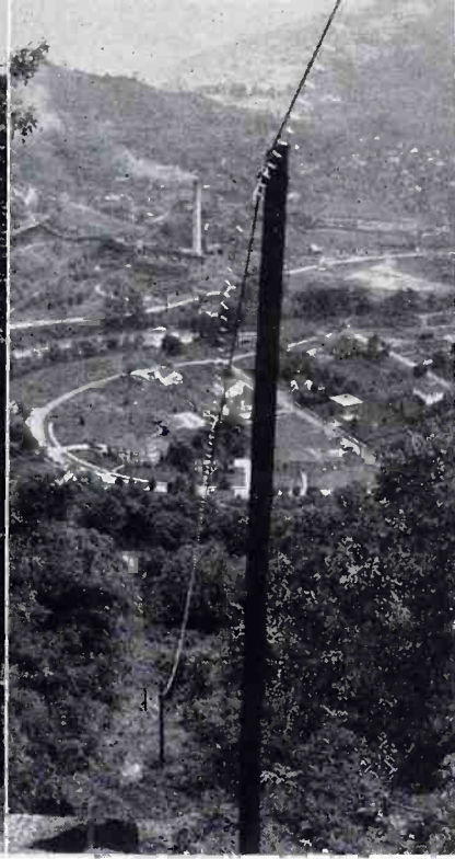
ABOVE: At Hazard, Ky., three antennas 1,000 ft. above the town pick up WSAZ-TV, WLW-TV, and WCPO-TV. Using amplifiers at the tower and along the 3,000-ft. Gonset-wire lead down the valley, signals are carried to a cable run on the power company's poles. Charges are $150 to $175, plus $4 to $6 for monthly service.
