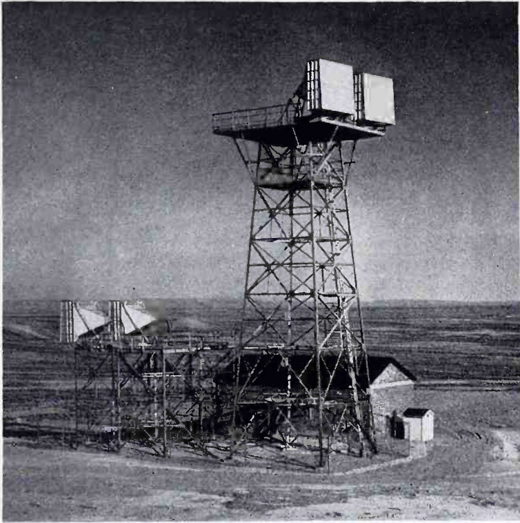
FIG. 3. TOWER AT CRESTON, WYOMING. NOTE DIFFERENT ANTENNA LEVELS. FIG. 4. A RELAY STATION IN THE SIERRA-NEVADA MOUNTAINS
