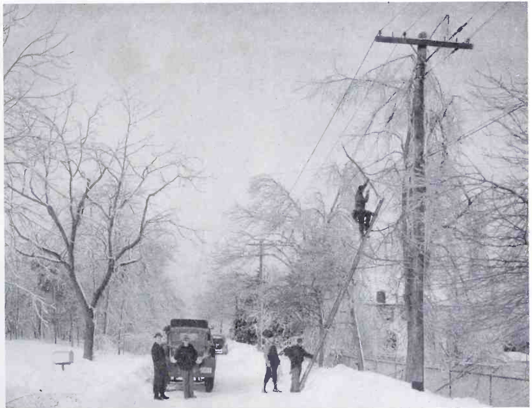
RADIO DISPATCHING ELIMINATES THE NEED OF RETURNING TO HEADQUARTERS FOR NEW ORDERS
