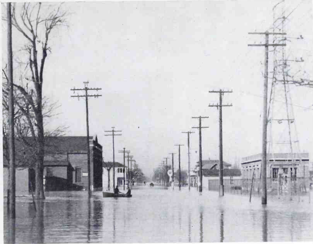
RADIO SPEEDS RESTORATION OF NORMAL SERVICE AFTER FLOOD WATERS SUBSIDE
