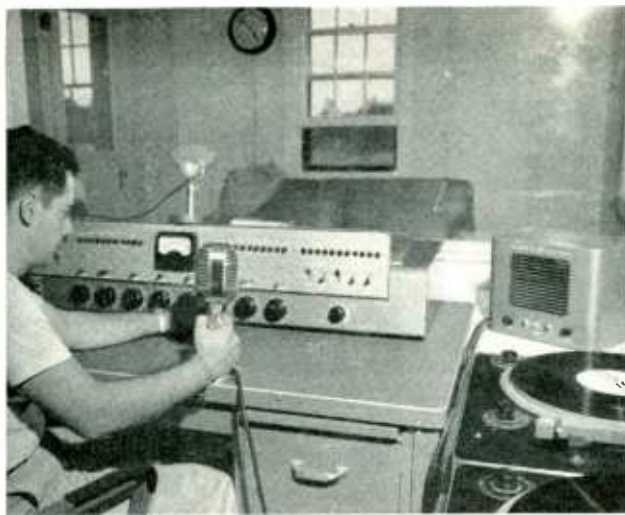
FIG. 12. Each station has a control console and turntables
