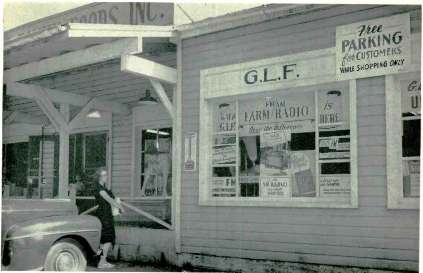
GLF stores are doing a job on FM set sales, installation, and service in rural areas equalled in few metropolitan centers. This is an important element of promotion
