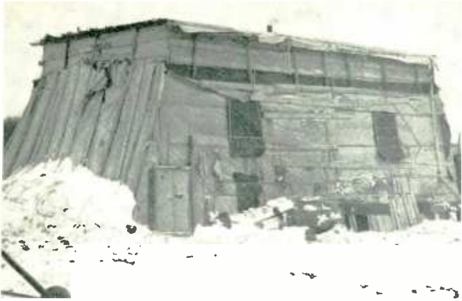
FIG. 1. View of the Wethersfield station shows winter construction methods. FIG. 2. Wraps were removed when heat was installed
