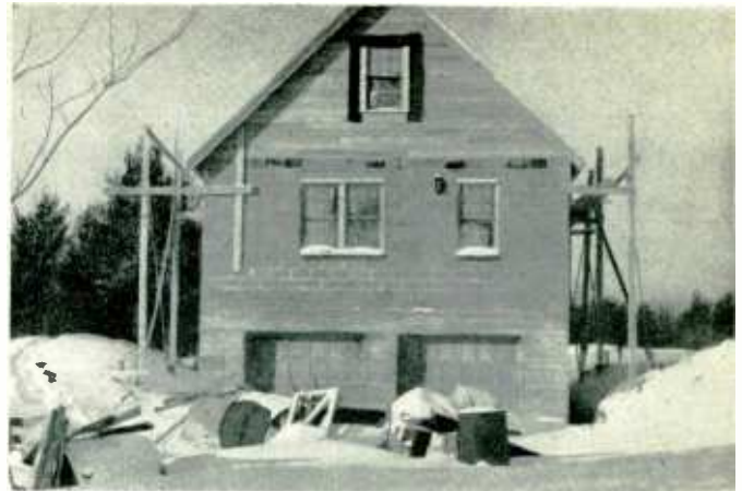
FIG. 1. View of the Wethersfield station shows winter construction methods. FIG. 2. Wraps were removed when heat was installed
