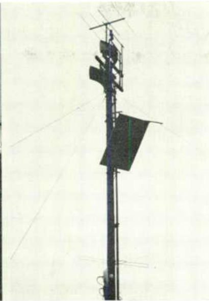
Fig. 5. At Oxford relay, microwave transmitter and face-up parabola are in cubicle at base of pole. Fig. 6. WABD receiving antenna at top, relay reflector below. Other gear belongs to Raytheon. Fig. 7. Receiver and controls at Oxford Hill
