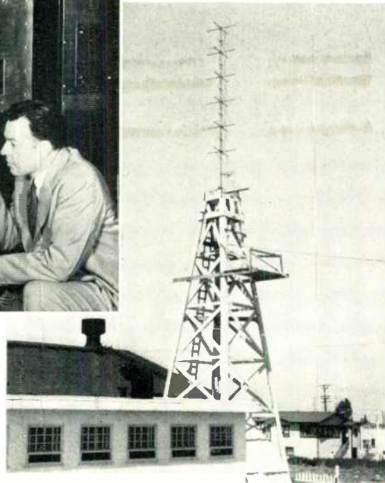
FIG. 1, ABOVE: JACK MCCULLOUGH, LEFT, AND BILL EITEL, WITH ONE OF THE NEW 3X12500A3 TRIODES. BELOW: 6-BAY TURNSTILE ON THE EIMAC PLANT AT SAN BRUNO, NOW SET UP FOR TEMPORARY USE
