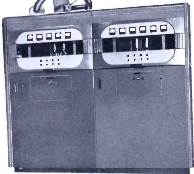
Collins 733A 3 kw FM Transmitter
