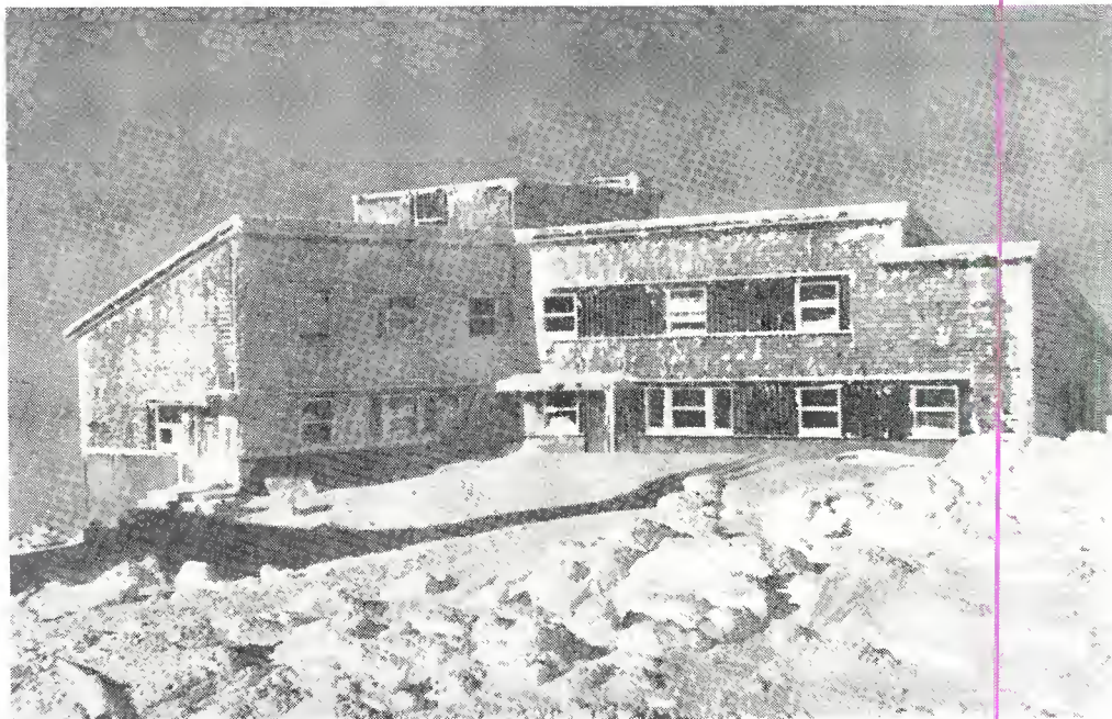
FIG. 1. THE 75-MC. RELAY ANTENNA IS INSIDE THE YANKEE NETWORK BUILDING
