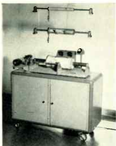
Alden Universal Scanner transmitting 18 inch copy with pre-loaded drums ready for immediate change to 4.1 inch or 8.2 inch copy transmission.
