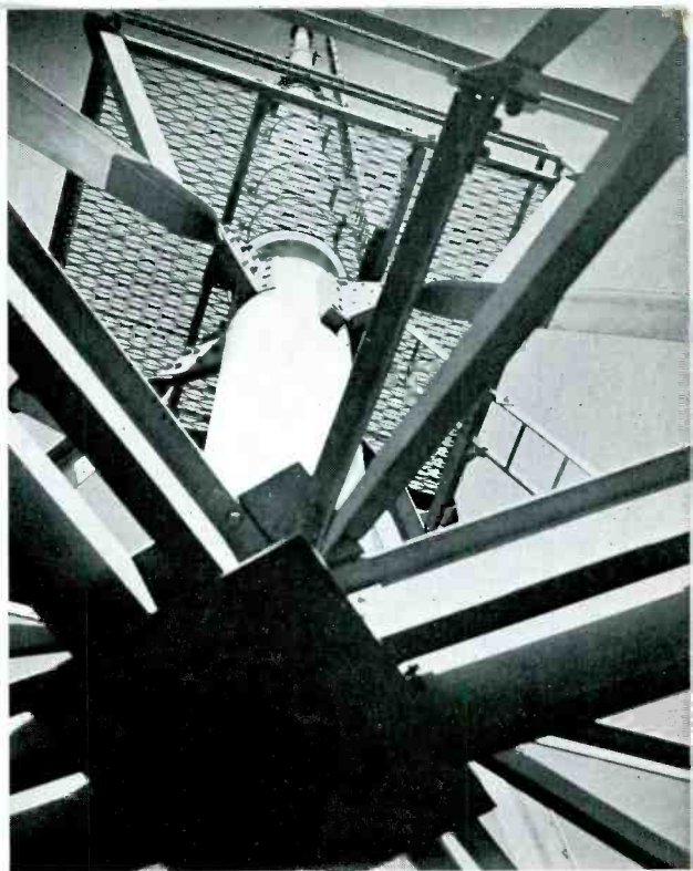
FIG. 6, LEFT: WITH THE BOTTOM SECTION IN PLACE, THE SECOND SECTION WAS LOWERED INTO PLACE AND WELDED TO THE FIRST. THE PIPE SCAFFOLDING WAS USED TO SUPPORT THE SECTIONS UNTIL THEY WERE WELDED. FIG. 7, RIGHT: LOOKING UP THE MAST AFTER COMPLETION
