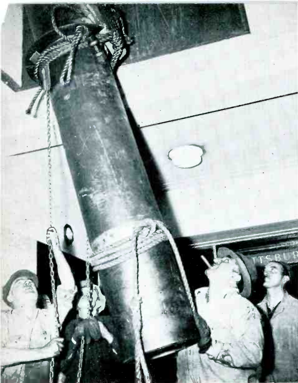
FIG. 4, LEFT: THE BOTTOM OR SOCKET SECTION OF THE FM ANTENNA BEING HOISTED FROM THE 58TH TO THE 60TH FLOOR. FIG. 5, RIGHT: THE NEXT STEP WAS TO RAISE IT TO THE ROOF OF THE TANK HOUSE, AND THEN TO THE SUPPORTING BASE. THIS MAST SECTION WEIGHS 2,200 LBS.
