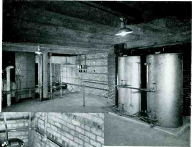
FIG. 9. CONSTANT CIRCULATION OF WATER FOR COOLING PURPOSES IS A VITAL NEED. FOR SAFETY, DUAL WATER PUMPS ARE PROVIDED, EITHER ONE OF WHICH CAN KEEP THE WATER FLOWING
