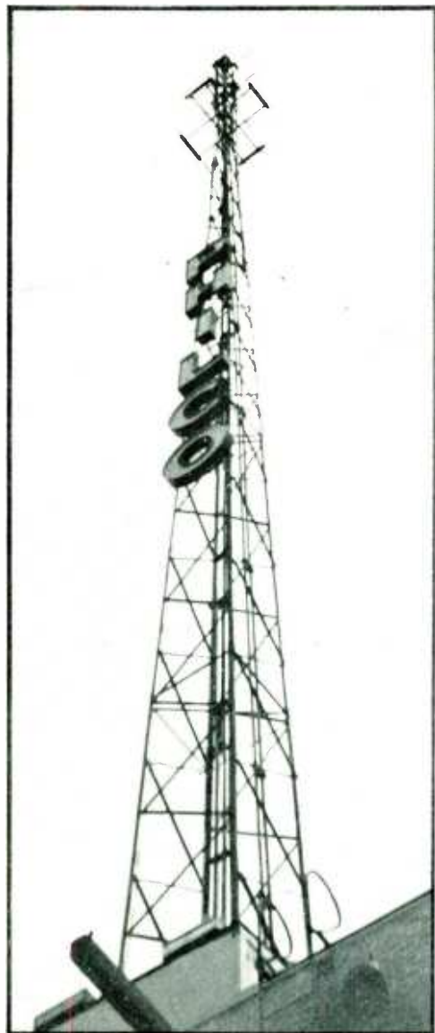
FIG. 3. MAIN STATION ANTENNA FOR VIDEO AND AUDIO SIGNALS, ATOP PHILCO FACTORY
