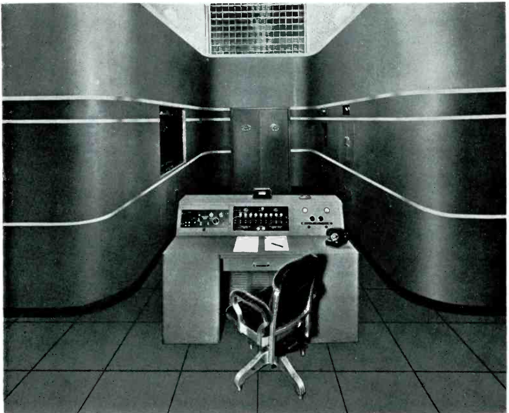
CONTROL DESK AND 50-KW. R.E.L. AMPLIFIER — THE WORLD'S FIRST 50-KW. F-M STATION
