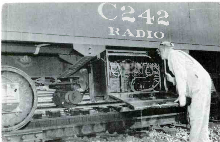
FIG. 1. VIEW OF THE 32-VOLT BATTERY COMPARTMENT AND GENERATOR
