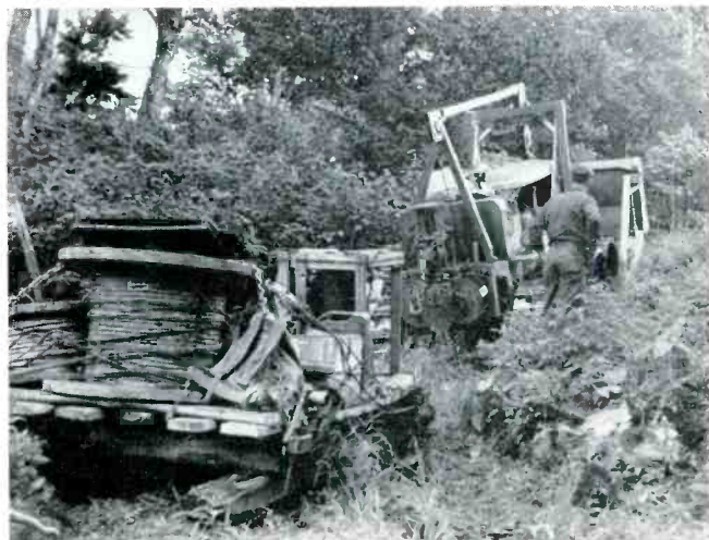
FIG. 3. EQUIPMENT BEING BROUGHT TO THE MOUNTAIN TOP BY TRACTOR
