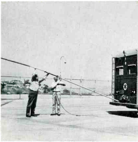
FIG. 7, ABOVE: MAST IS ASSEMBLED FROM SECTIONS CARRIED IN LONG COMPARTMENT UNDER THE TRUCK. TWO MEN CAN PUT IT TOGETHER QUICKLY. FIG. 8, RIGHT: SIMPLE FIXTURES ON THE TRUCK HOLD THE ANTENNA SECURELY. THE LEAD PLUGS INTO A COAXIAL CONNECTOR
