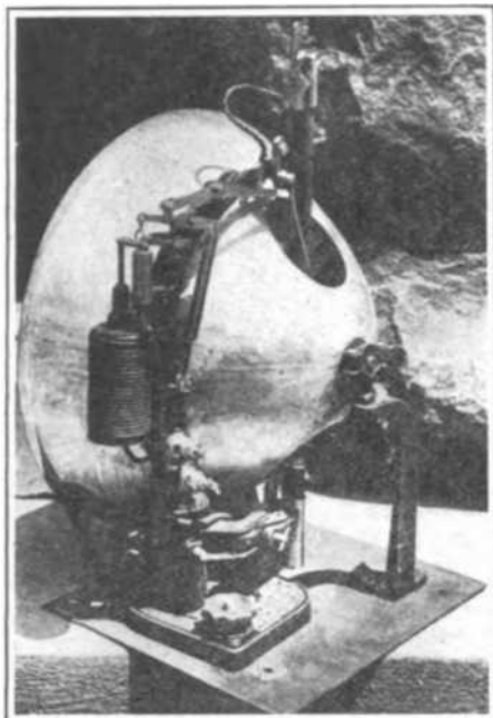
Modified locomotive headlight used to illuminate convention hall
