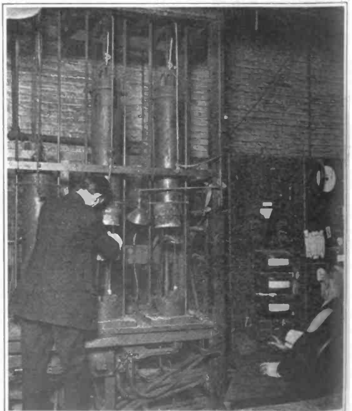
Putting a tungsten slug into treating "bottle" where an electric current is passed through it in a hydrogen atmosphere. This makes the tungsten a degree stronger
