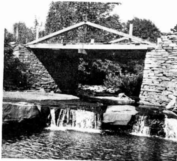
Fig. 3. The use of the roof truss in bridge construction. This very simple application of the truss is described in this article
