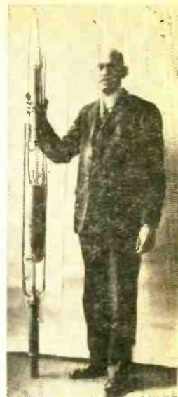
Top—At Clark University in 1924, Goddard lectures on how man eventually might reach Moon. Right—Goddard with his liquid-fueled rocket: motor is at base, fuel tanks are above it.
