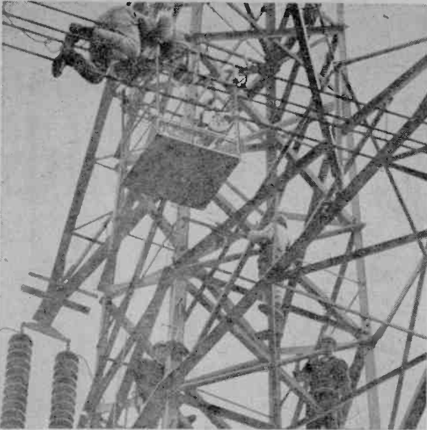
Cables Harry's sitting on carry 400,000, but Harry pays them no-never-mind. Explanation is that wire-mesh-and-cotton suit he's wearing places him at same 400,000-V potential as line. Remainder of team look on from safety of pylon as Harry juggles his equipment trolley into place.
