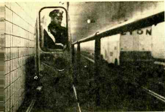
Gasoline-powered vehicles, 20 inches wide and guided by a unique single-rail system on a catwalk, enables tunnel police to speed to any part of Lincoln's South Tube.
