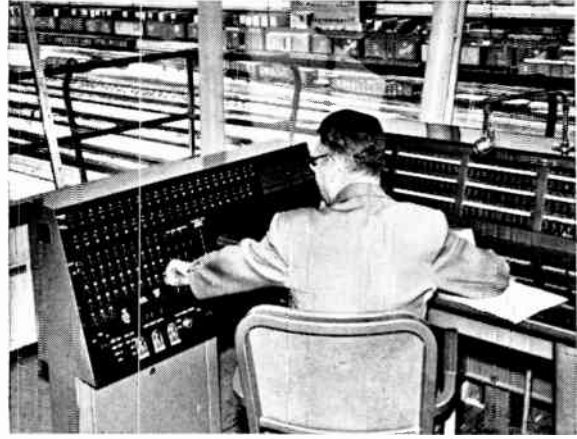
Analog computer panel (left) made by General Railway Signal and various electronic units (right) from Union Switch and Signal play key roles as railroad men . . .
