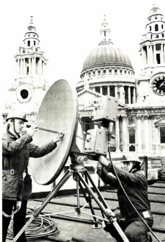
Royal dish. British Telecom technicians set up microwave dish on building in St. Paul's Churchyard in London to transmit TV pictures of last summer's royal wedding.
