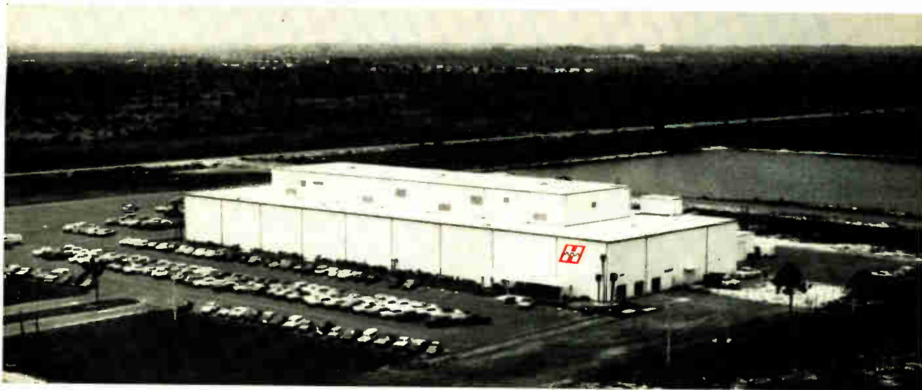
HARRIS SEMICONDUCTOR . . . a new name and a new IC manufacturing facility with approximately 113,000 sq. ft. of the latest innovations in wafer manufacturing and development. (Located in Melbourne, Fla.)
