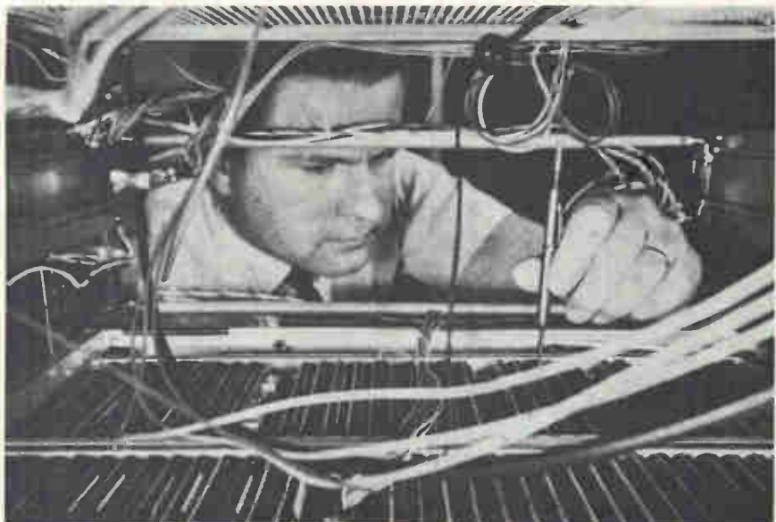
Logical starting point. Comsat technician checks reallocation-logic section of an experimental time-division multiple-access system; work on this project will continue at the company's new lab.
