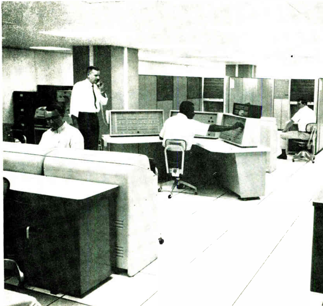
Cortex. View toward the two ITT 7300 message processors that are the nerve center of State's communications center in Washington.
