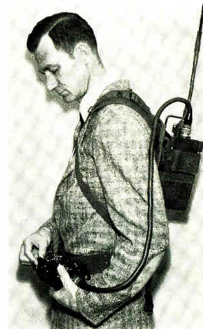
Tune in. Backpack loran tells a rifleman where he is.
