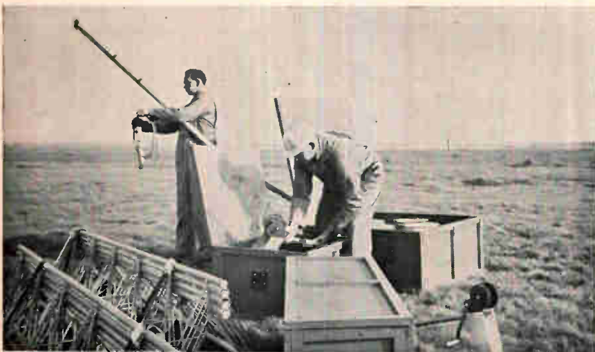
Skywave high-frequency antenna developed by Granger Associates fits into a 90-cubic foot package and can be assembled in two hours by five men. The antenna bounces signals off the ionosphere, thus skirting the problem of attenuation that's caused by dense jungle.
