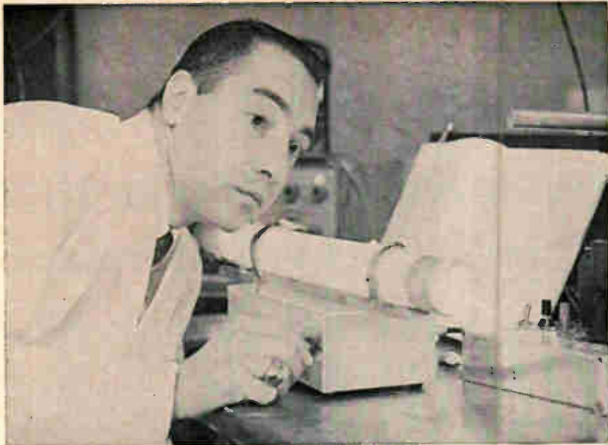
Richard Zipin of the Sheffield Corp. is one of many research associates from industry who work at the National Bureau of Standards. Here, Zipin adjusts a laser used in making interferometric measurements of length.
