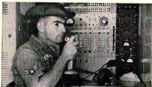
Air commandos at home base will use this AN/TSC-15, an h-f/a-m/ssb radio, with power up to 900 watts, to talk with their men in enemy territory.
