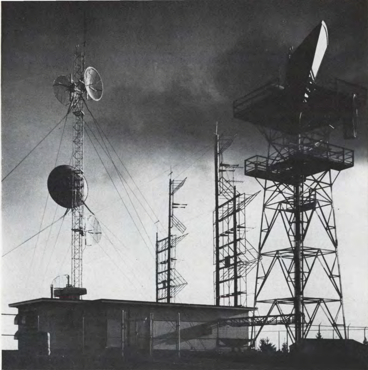
Microwave repeater system for television transmission, similar to the system shown operating in Canada, will be supplied to Yugoslavia by the General Telephone & Electronics Corp.'s Italian subsidiary, Marelli Lenkurt S.p.A. The equipment, costing $1 million, will consist of four microwave links operating over 600 miles.
