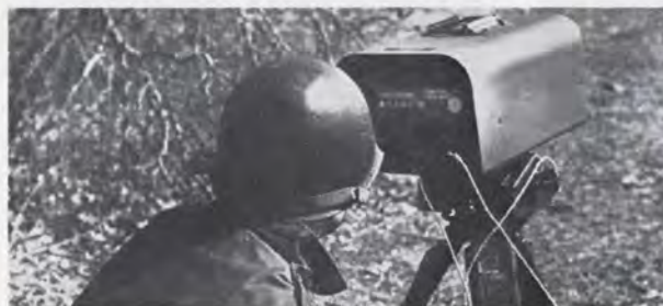
Laser range finder developed for the Army by RCA uses pulsed laser and digital readout. Integrated sighting and receiving telescope developed by Bausch & Lomb, Inc., transmits light to photo detector and protects the user's eyes. The Army is testing several laser range finders for possible field use.
