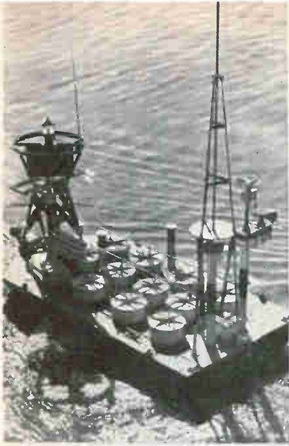
NOMAD BUOY. Martin Co.'s atomic-powered meteorological reporting system has just been installed in the Gulf of Mexico
