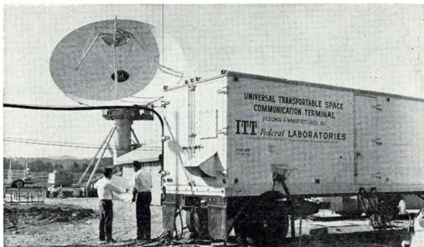
TRANSPORTABLE STATION at Raisting, Bavaria, operates at both Telstar and Relay satellite frequencies. The American-made equipment was installed by Standard Elektrik Lorenz, ITT affiliate
