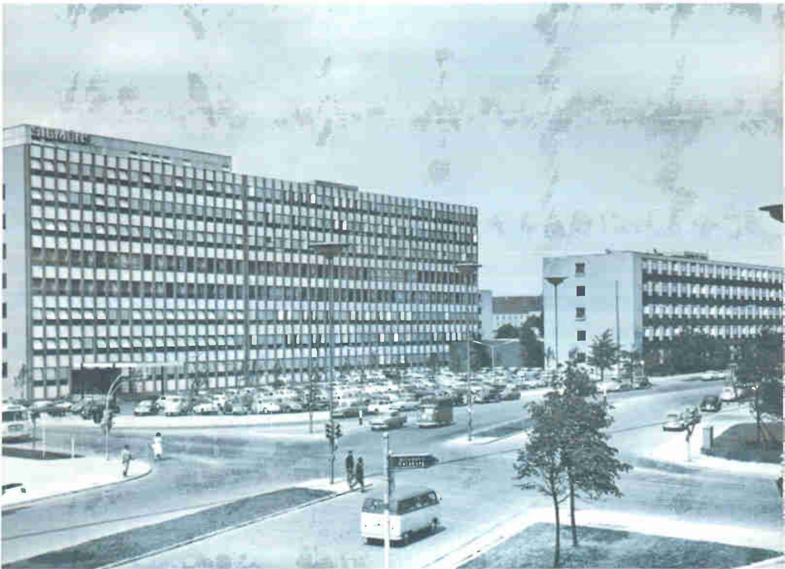
Siemens Components Center, Munich—Main Offices, Research, Manufacturing and Sales
