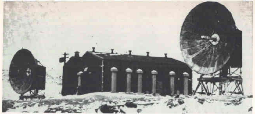
TROPO terminal in Greenland is part of 240-channel Dew East network linking northeast North America with Greenland and Iceland
