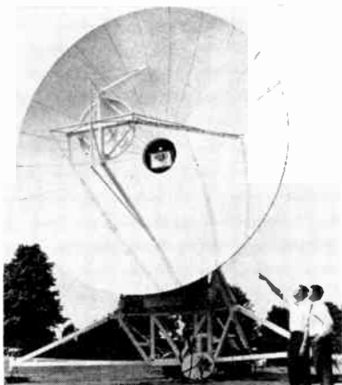
STEERABLE 30-foot antenna developed by Antenna Systems, Inc., for ITT Federal Labs can be transported on two trailers or by air carriers. ITT will use the first one for the Project Relay satellite program
