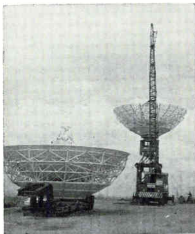
C-BAND ANTENNA, 30 feet in diameter on truck (left) waits for shipment as the 40-foot L/X-band antenna is hoisted to turntable at radar test range
