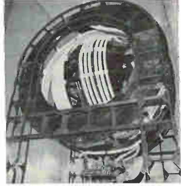
Enormous variometer coil for inductance to tune the antenna system through a range of 14 to 30 KC . . . very low frequency. These VLF radio waves penetrate the depths of the sea to submerged submarines.
