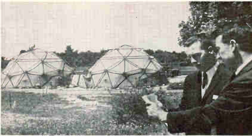
COLLAPSIBLE HUTS house electronic equipment. These two huts are part of a test installation at Watertown, N. Y.
