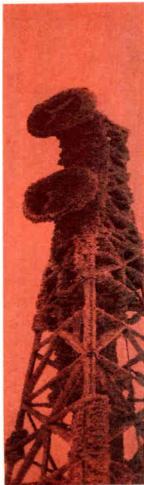
SOUTHERNMOST TIPS of Ontario are at the level of northern California but the Canadian climate is not always as warm. This CNT microwave tower in Newfoundland beams its signals across the Cabot Strait to the mainland even in a storm
