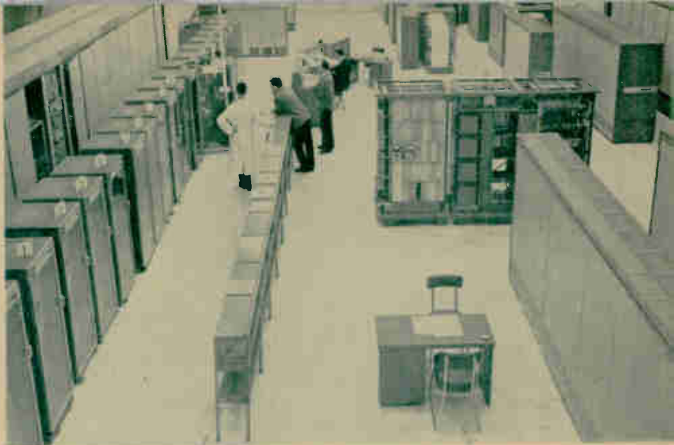
Bull computer installation in Paris
