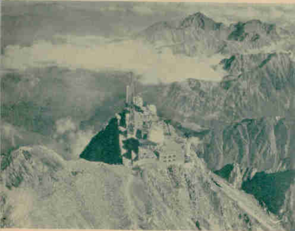
TRT's antenna on the Pic de Midi de Bigorre in the Pyrenees is the starting point for a tropo scatter system that relays French tv programs to Algeria by way of Mallorca
