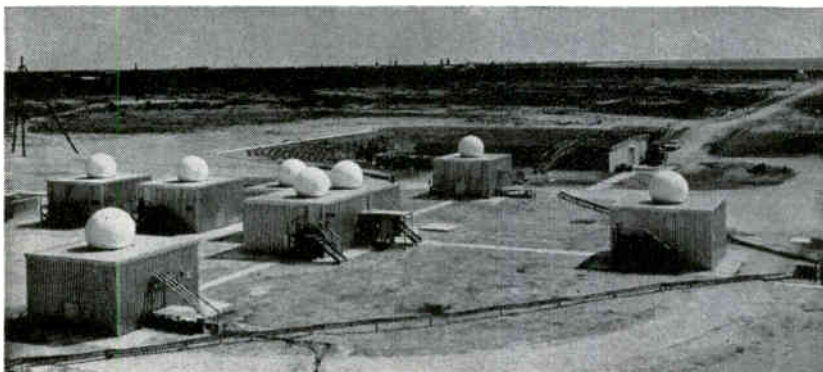
White radomes enclose precision antennas of Convair Azusa Mark II system which enable USAF to track missiles with accuracy of a few feet at hundreds of miles
