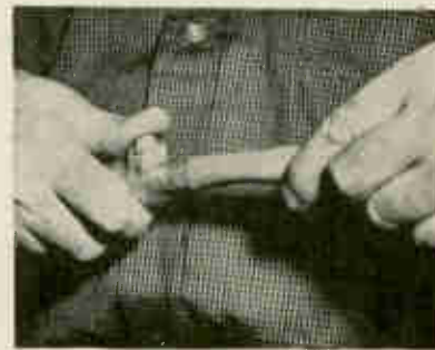
Blowing wad and cord through
