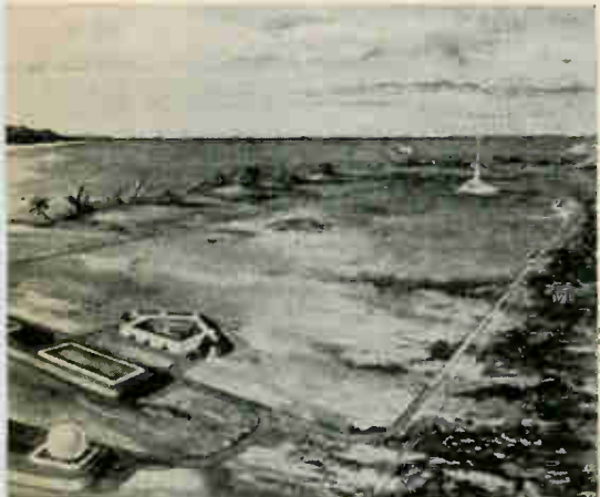
Portion of site shows target tracking, discrimination, Zeus tracking radars and (rear) Zeus being launched
