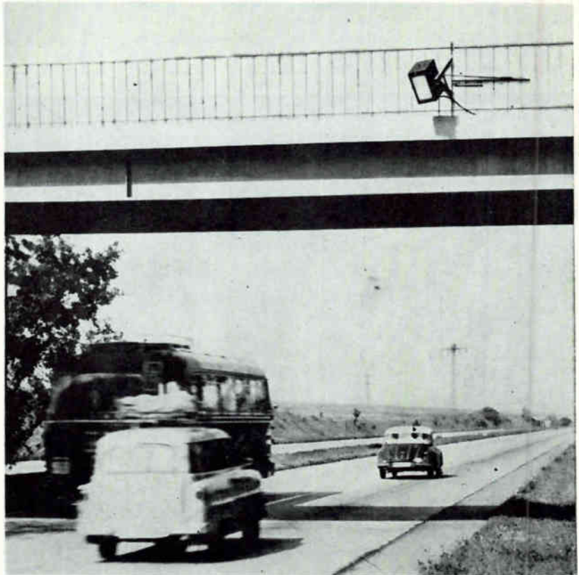
Traffic analyzer positioned on highway overpass. Note tubular antenna
