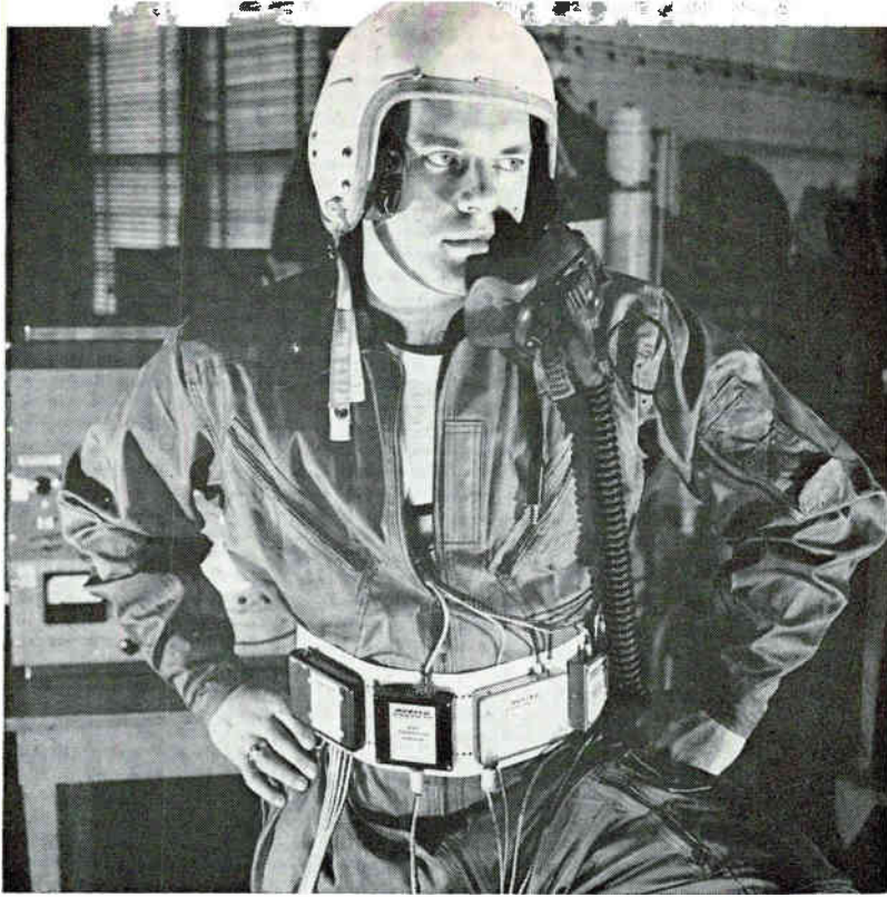
Miniaturized instruments accomplish simultaneous recording of body functions for Boeing bioscientists
