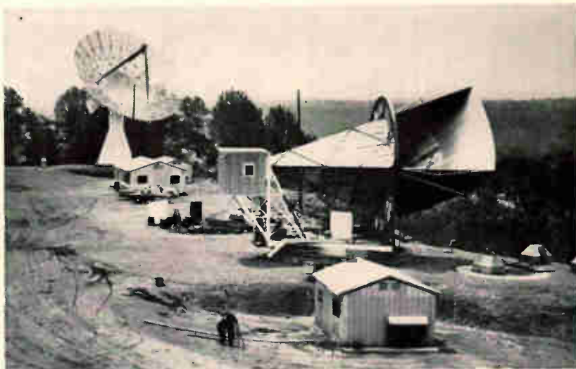
Installations like this Project Echo transmitter and receiver at Bell Labs' Holmdel, N. J. site will figure in future earth to satellite systems
