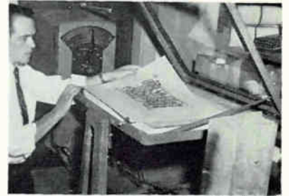
Master is photographically reduced to actual board size
