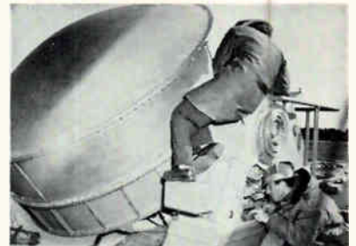
Weldment serves as tracking radar antenna mount
