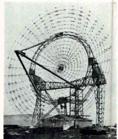
Stanford Research will study the aurora for ARDC with this spider-web, 142-ft radiotelescope in Scotland
