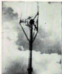
Surveillance radar towers on the DEW line. Designed for hurricane force winds and heavy ice and snow loads. These are some of more than 1000 radar towers built by Dresser-Ideco for the nation's aircraft warning system.
