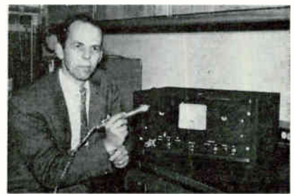
Close-up of central unit and probe
