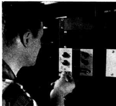
Technician inserts amplifiers in rack-mounting assembly
